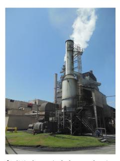
conducted, it was concluded that the development and installation of a CHP plant to include a combustion turbine generator and HRSG was a viable economic, technical and environmental solution.
