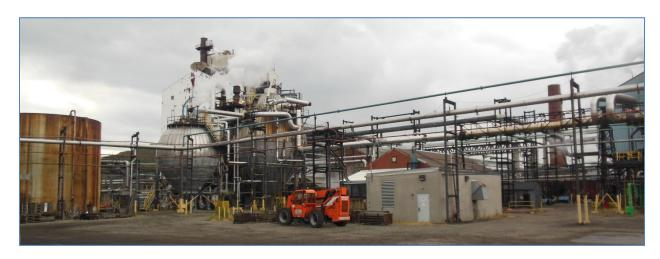
The configurations evaluated included new and secondary market (refurbished used) equipment including GE Frame 6 and LM2500 combustion turbines in simple and combined cycle configuration. The configuration selected as optimum was a combined cycle configuration with two Frame 6 combustion turbines, a new steam turbine, and the existing steam turbine.
